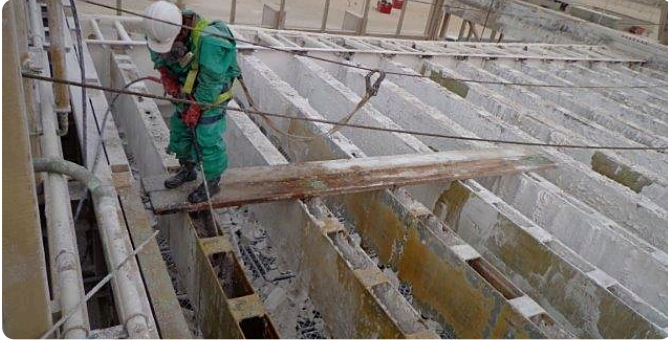
Fill replacement inside an operating tower
