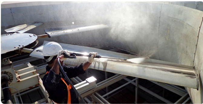
Mechanical equipment alignment
