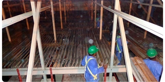
Tower internals during rehabilitation
