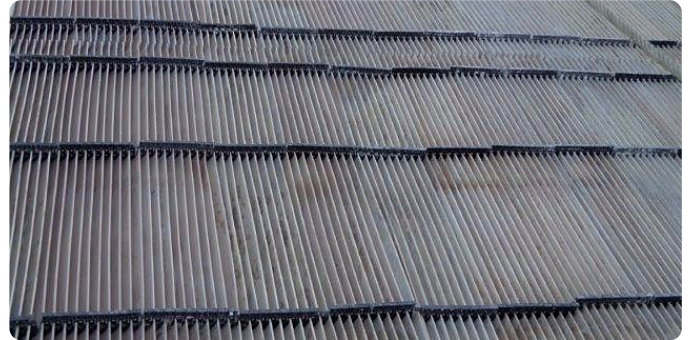
After hydro-jet cleaning
